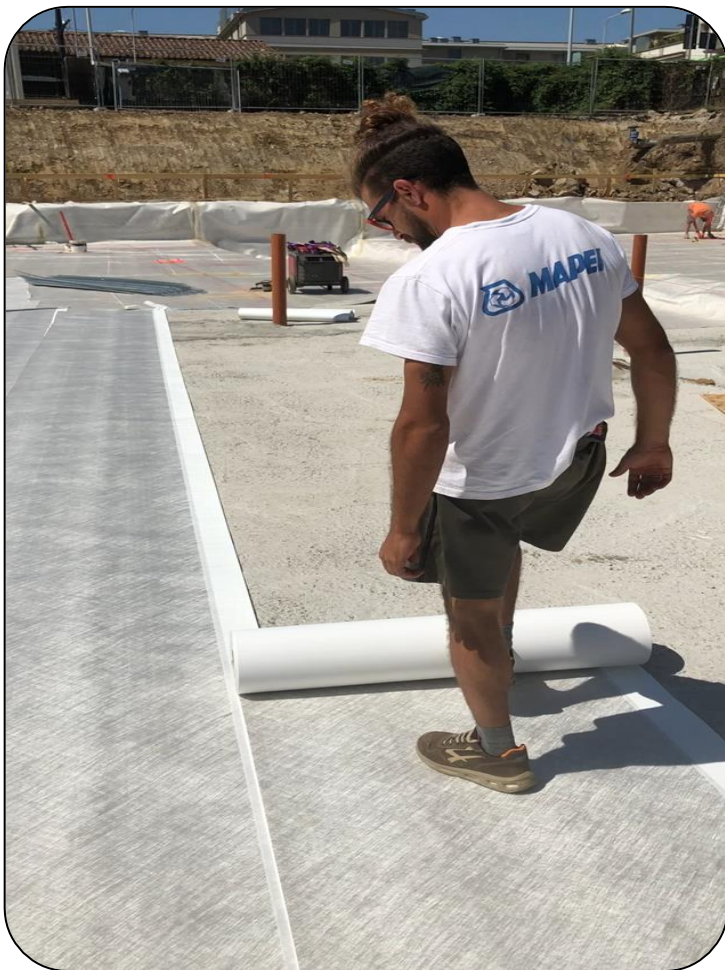
MEMBRANE FULLY BONDED
