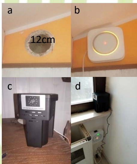
Figure 1. Respire Remediation System: a) SNAP must be installed on a wall in a 12 cm diameter hole that communicates directly with the outside; b) SNAP with working fan, the yellow light indicates that indoor radon concentration is below the reference level of 300 Bq/m 3 ; c) RD200M connected via Bluetooth with the SNAP; d) complete Respire Remediation System mounted in a school at Celleno municipality.
